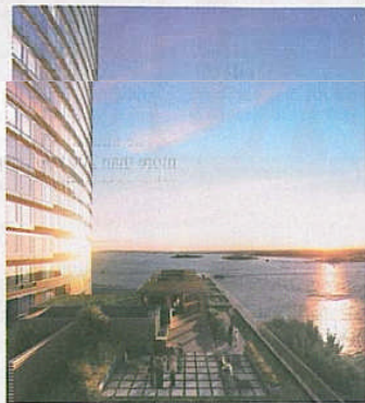
The Visionaire in Battery Park City is one of the most technologically advanced residential buildings in the country.
