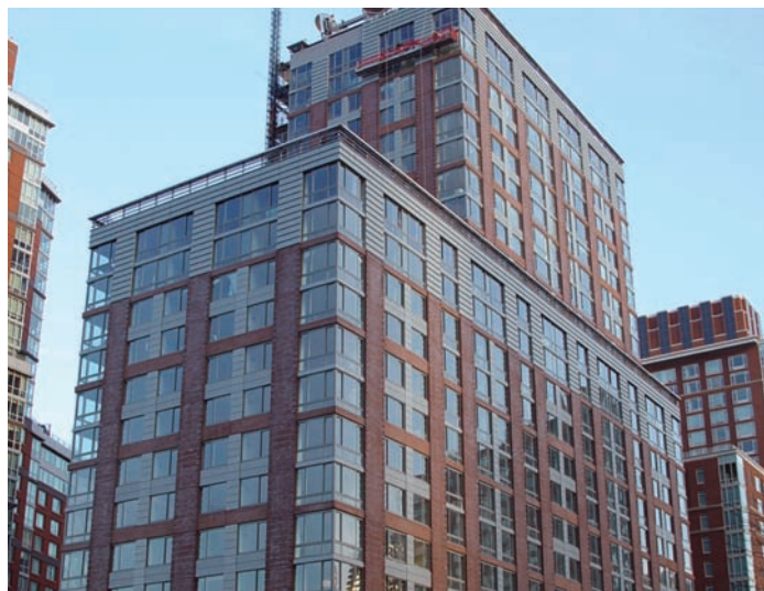
SECOND GENERATION: Roughly 8 percent of the cost of building The Verdesian went toward green features. About twice that was spent on the building’s predecessor, The Solaire.
