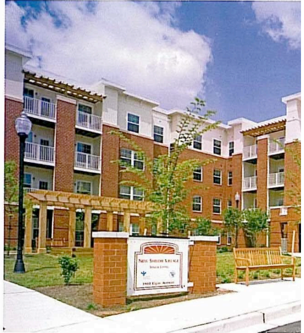
Enterprise Homes included energy-efficient features and used low-volatile-organic-compound paints and sealants in the affordable rental homes at New Shiloh Village Senior Living in Baltimore. The development, which opened in 2007, was designed by Hord Coplan Macht of Baltimore.
